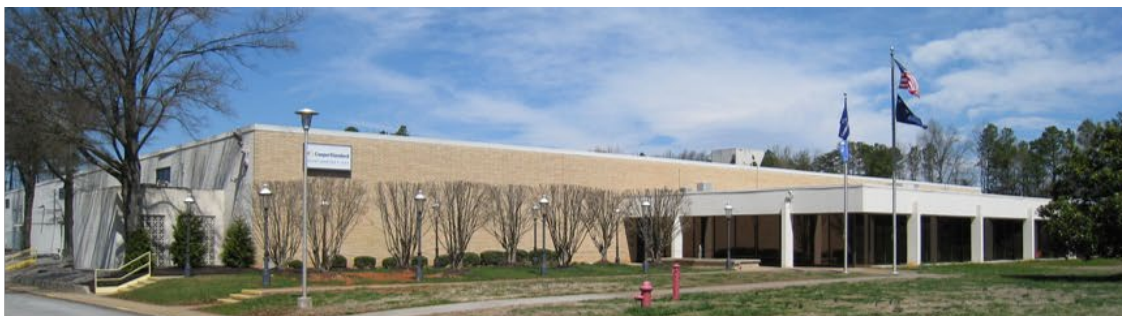
Spartanburg Plant Expansion Complete
